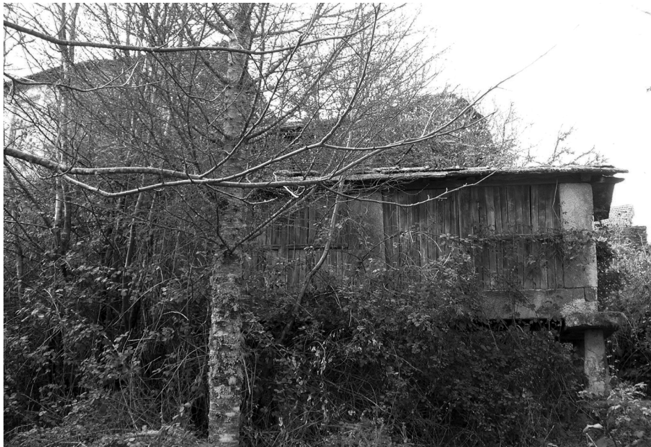
Figure 10. Ruined houses and granaries, concealed by overgrown vegetation, in Galicia (Spain).
