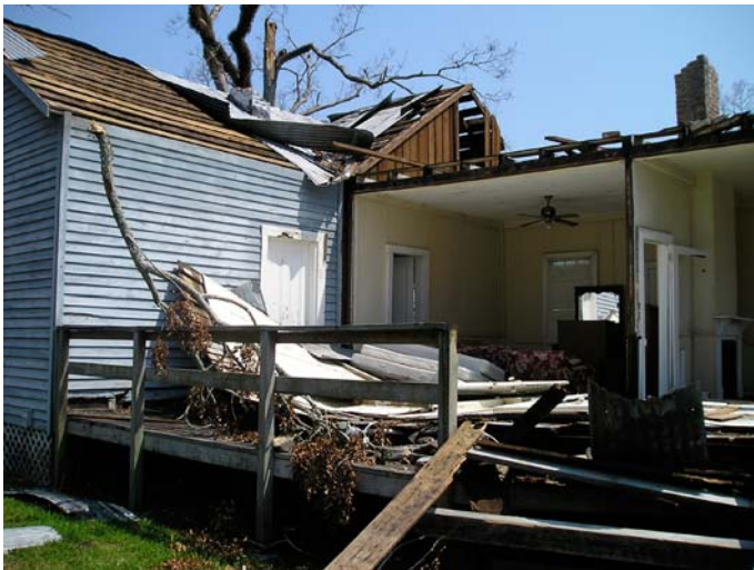
Figure 1. Ruins of a home in Bay St. Louis, Mississippi, September 2005. Source: Photo courtesy of Schomer
